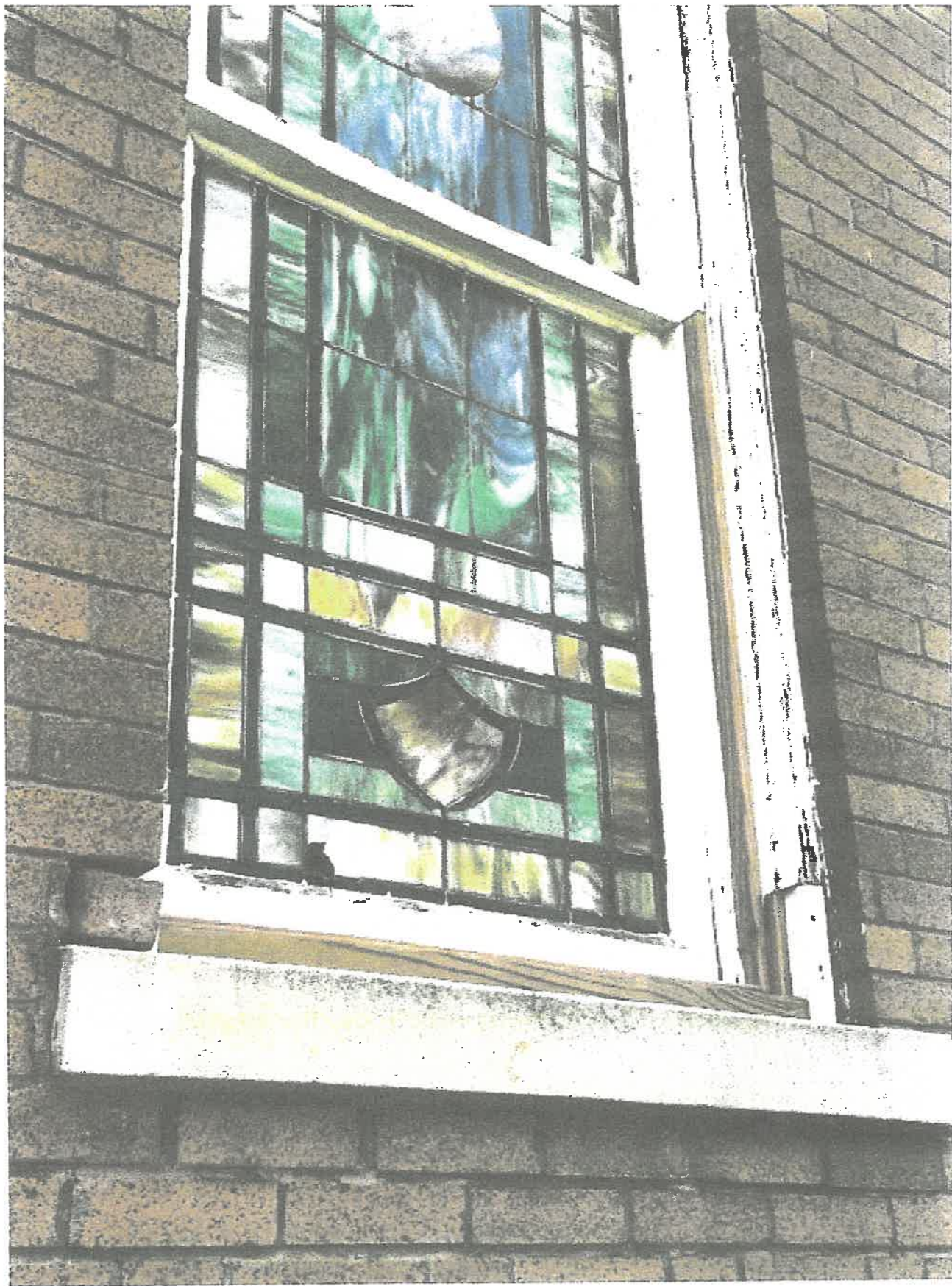
Bradberry NJB Window repair
